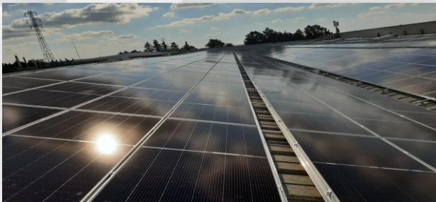
Tayeks Silivri - 2,187.30 kWp
