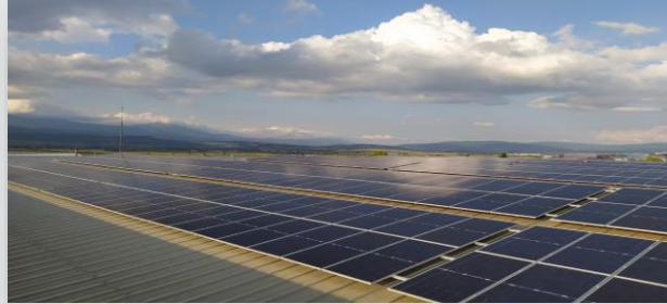
Tayeks Bolu - 2,073.22 kWp
